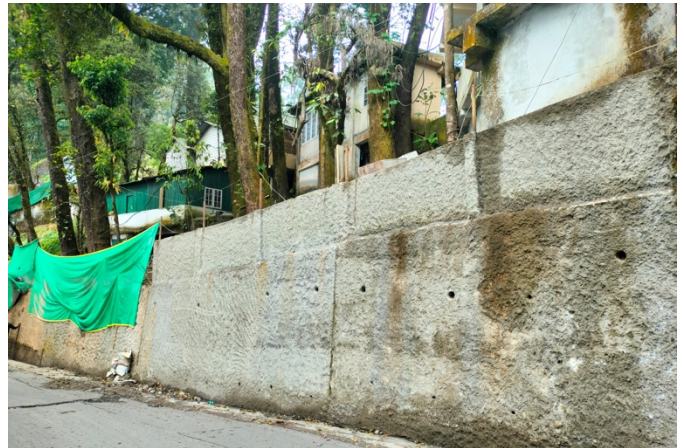
Wall below main gate
