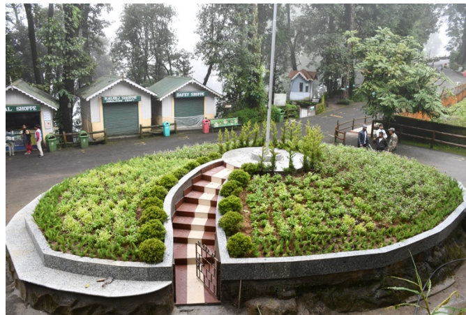
Construction of flag hoisting area
